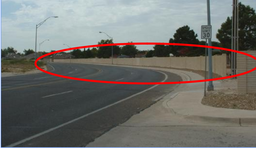
FIGURE 7.3a: Enhancing Perimeter Walls Hobbs Comprehensive Community Development Plan City of Hobbs, New Mexico
