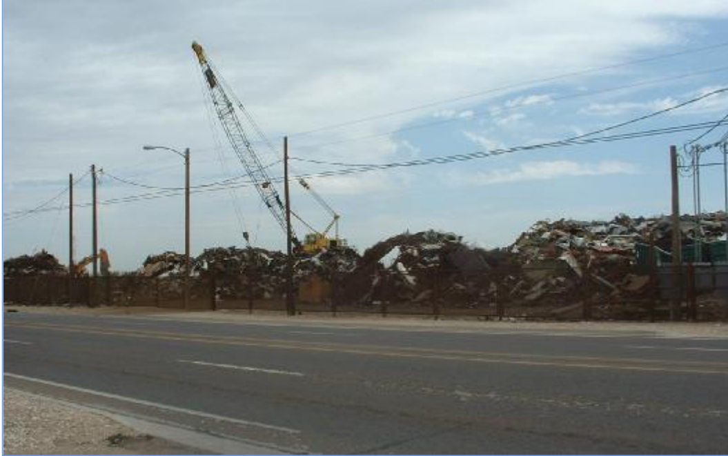
FIGURE 7.2b: Screening Unsightly Views Hobbs Comprehensive Community Development Plan City of Hobbs, New Mexico
